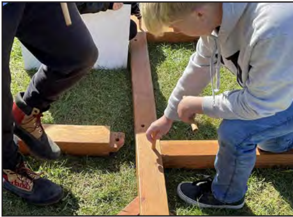
FFA member Owen Cipta inserts one of the wooden pins used to hold the post and beams in place. Photo provided by Robert Richards
