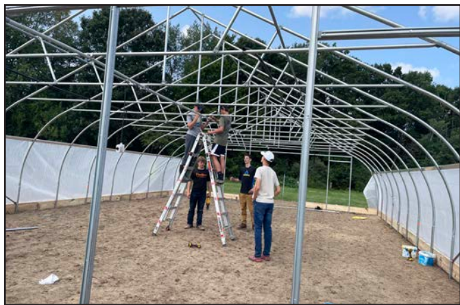
Agricultural, Construction, and FFA students installing the frame for the hoop house. Photo credit Joan Tucker
